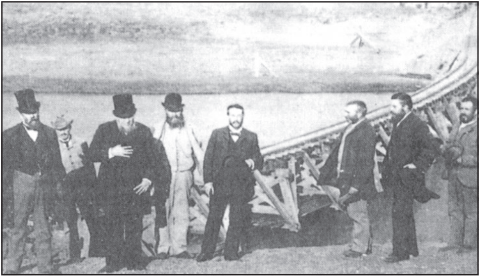
Illustration: In 1892 the railway bridge over the Vaal River at Vereeniging was taken into use. President Paul Kruger (third from left) and the entrepreneur Sammy Marks (third from right) at one point made plans to transport water in railway carriers to Johannesburg. 26
