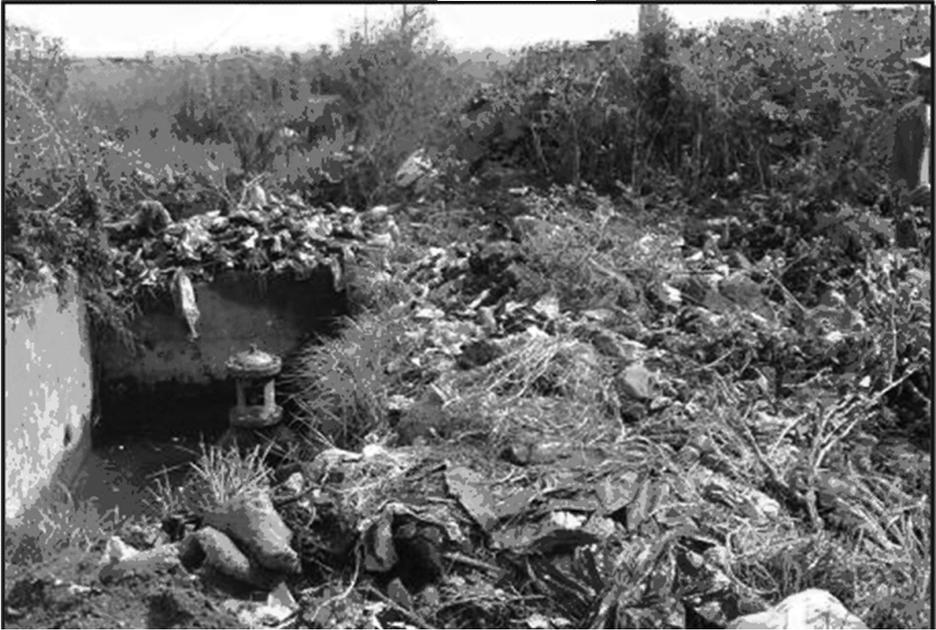
Figure 6: Identification of missing valve and chamber after cleaning
