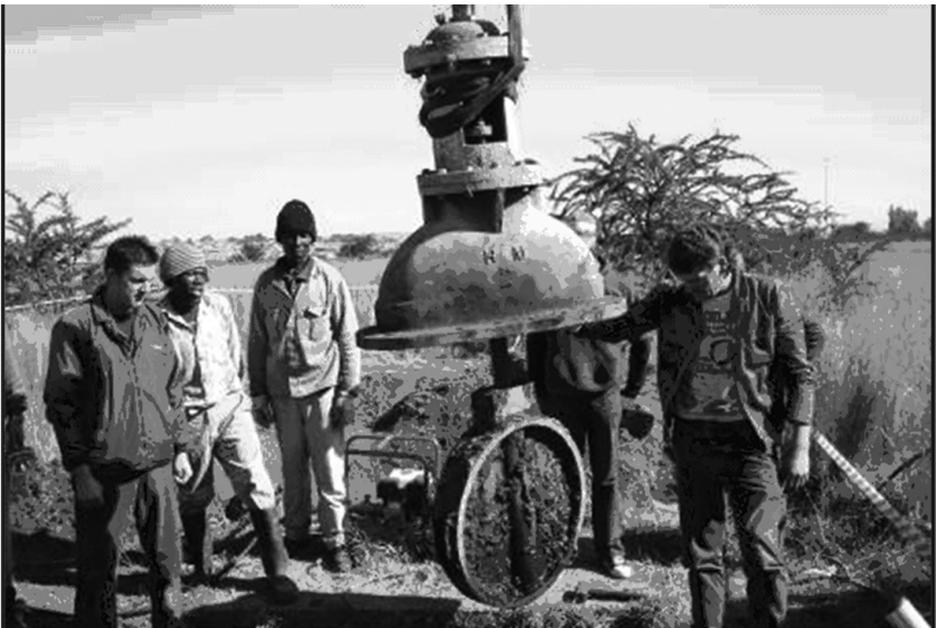
**Figure 7: Removal of valve body**
